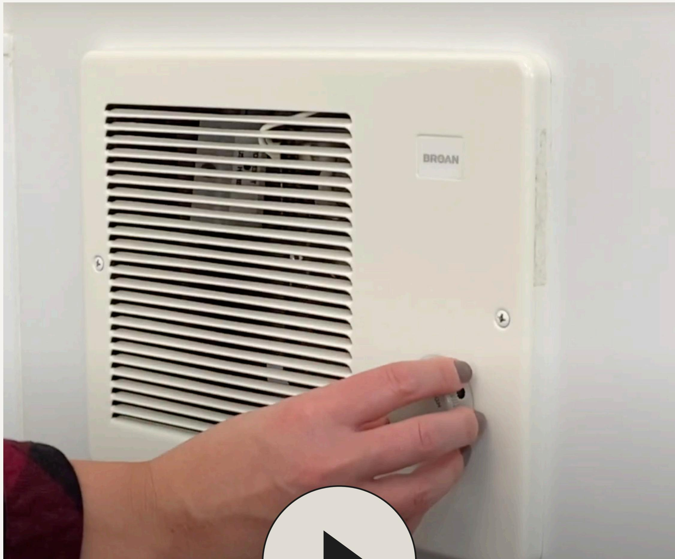
**To operate your wall heaters**, simply turn the thermostat dial to your desired temperature. On those chilly nights, we suggest closing the bedroom door with the heater kept on for the most warmth.
