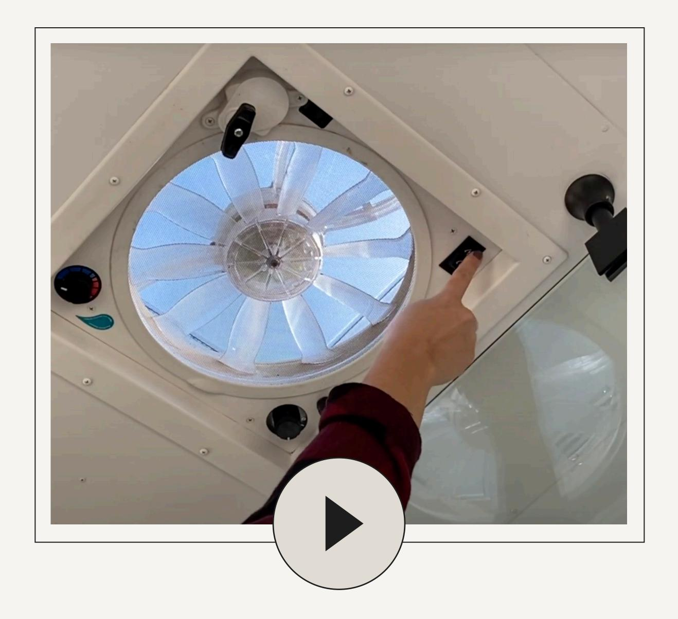
There is a fan in your suite bathroom. Your fan should remain in the **ON** position at all times. Fans will not operate and will close automatically if it's raining or if there is heavy dew.
