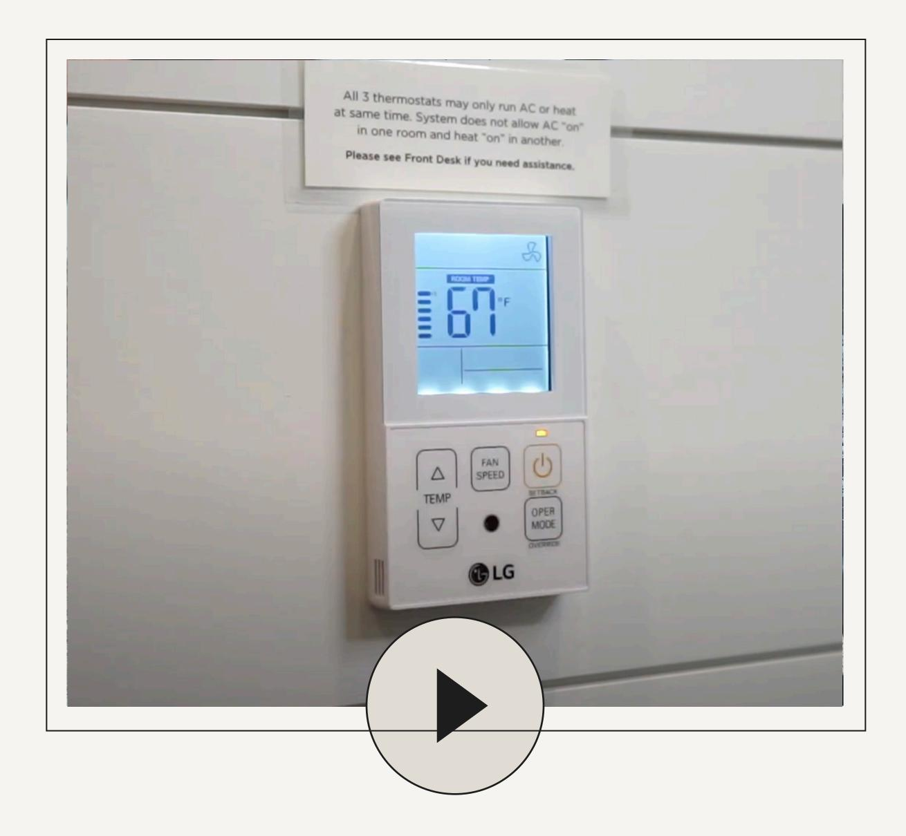
For air conditioning, locate the digital thermostat on the wall next to the door. To operate the thermostat, press the POWER button once to "wake it up". Then press the PROGRAM button. Press the MODE button to change the setting to COOL for Air Conditioning. Adjust the temperature with the up and down arrows to your desired level. To turn off the air conditioning, simply press the power button.
