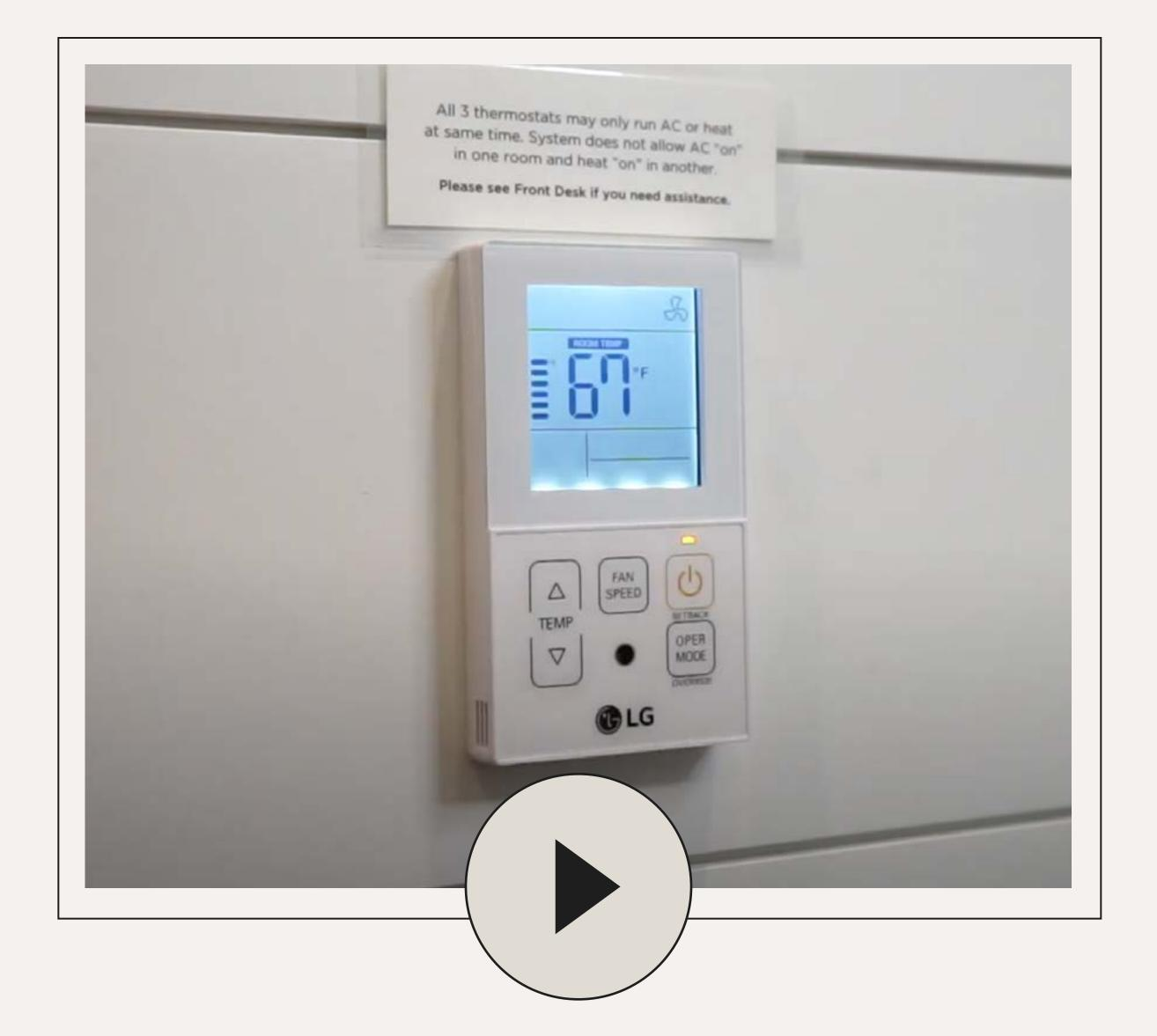
To operate the thermostat, press the large button once to "wake up" the thermostat. Use the large button to change setting to FAN or COOL for A/C, or HEAT. Adjust the temperature with the up and down arrows. To turn off, click the large button until the display shows OFF.
